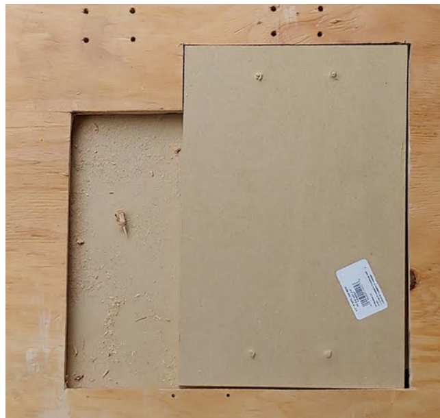
Figure 1. The open slot for the lock along the door.
